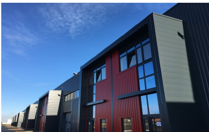
Eastern view of the Roméo business park in the Cargo area of Paris-Orly Airport ©Groupe ADP
