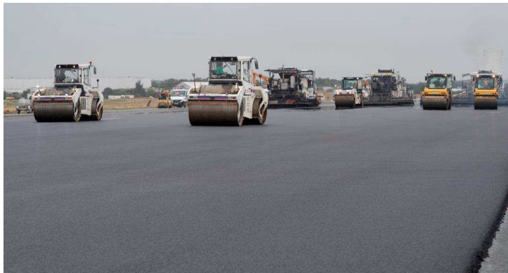
Renovation work on runway 4 in 2017 Photo Groupe ADP-Alain Leduc
