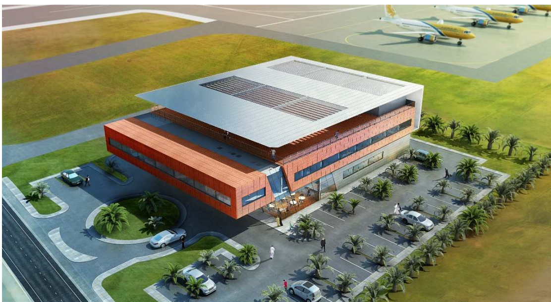
View of the new air traffic control centre at Bahrain International Airport © ADP Ingénierie
