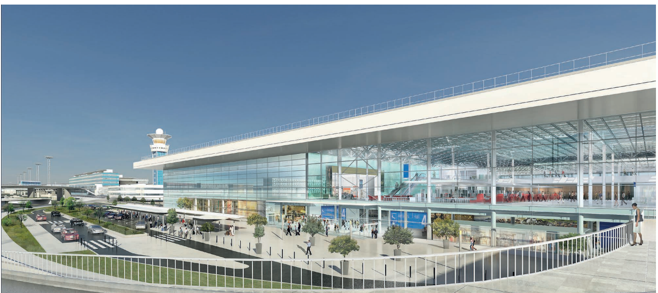
View of the outside of the future connecting building linking the South and West Terminals at Paris-Orly © Groupe ADP
