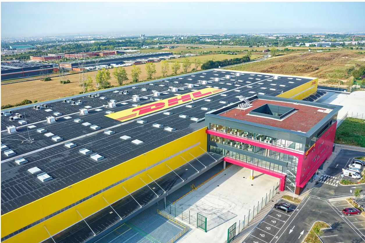
New logistic hub of DHL Express in the Cargo City of Paris-Charles de Gaulle airport © DHL Express
